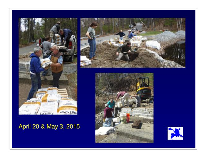
We've had a recurrent, small leak in the westerly side of the dam, resulting in sinkholes which have opened up early each spring over a number of years now. In 2015, it happened again, and this time we used a special clay - which expands when wet to form an impermeable barrier - to seal the channel. Here are volunteers at work making the repairs.
