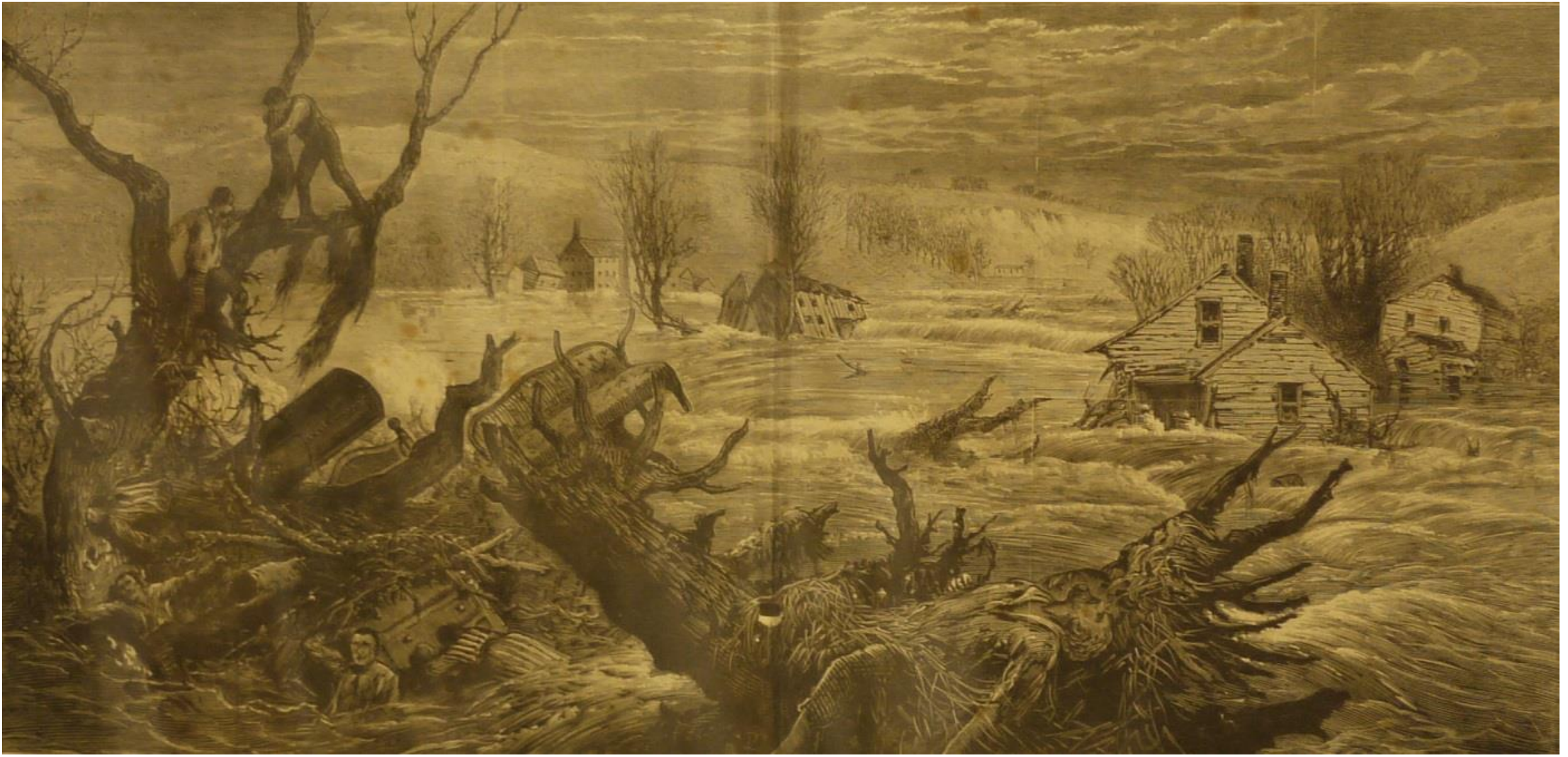
The Williamsburg Reservoir Dam Failure of 1874
