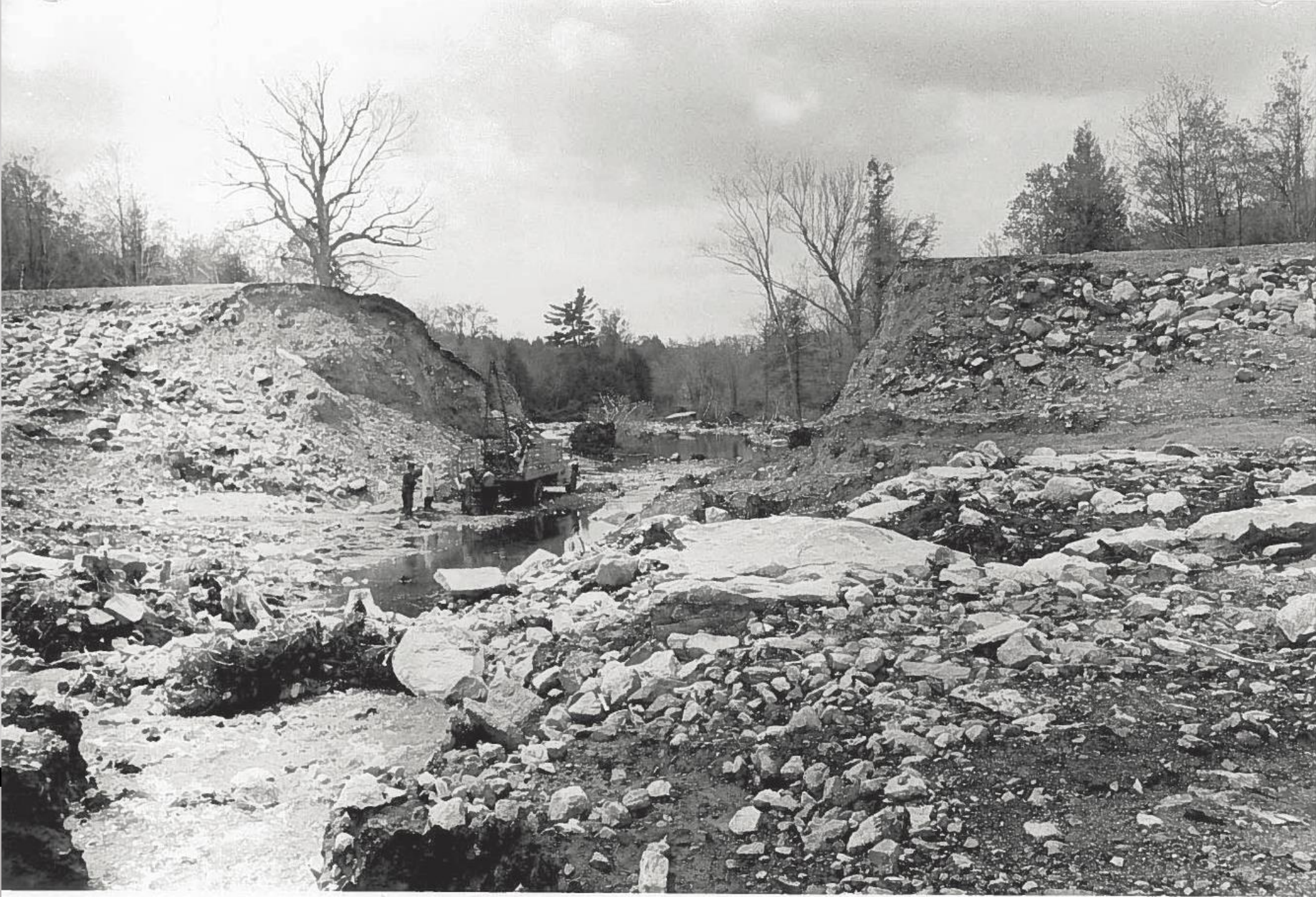
Lake Lee Dam after breach
