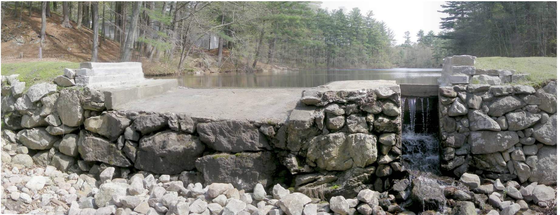
Photo 8 – Panoramic composite – Spillway, sluiceway, and plunge pool from downstream*
