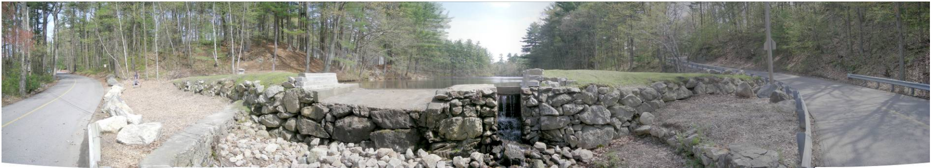
Photo 5 – Panoramic composite – Downstream face, spillway, and sluiceway from downstream*
