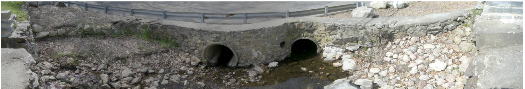
Photo 11 – Panoramic composite – Downstream part of plunge pool and culverts under Rattlesnake Hill Road, from spillway*
