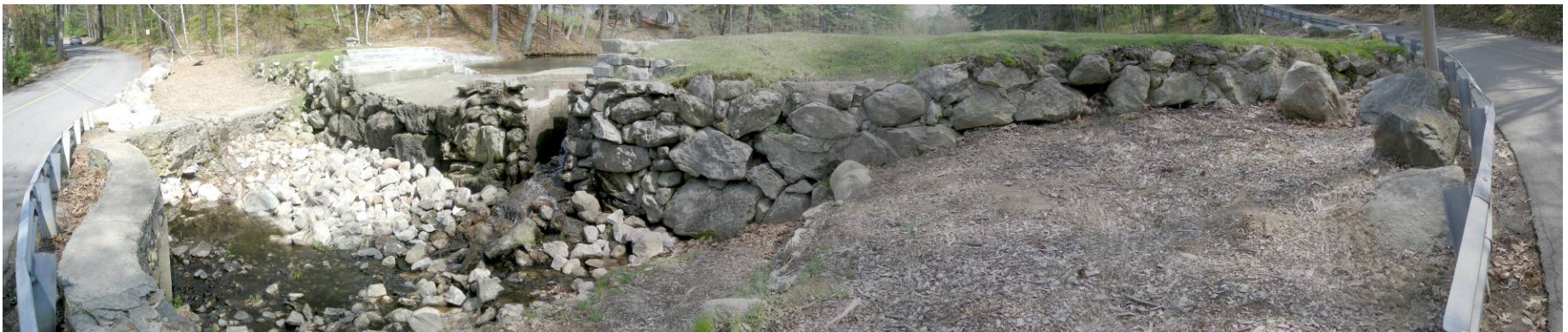
Photo 7 – Panoramic composite – Left downstream face, spillway, and plunge pool from downstream*
