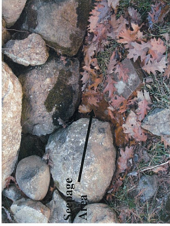
Photo 16 – Seepage on right side, at toe
