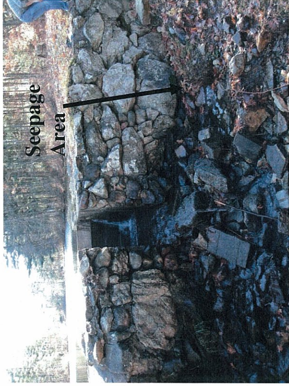
Photo 15 Sluiceway and seepage area on left side
