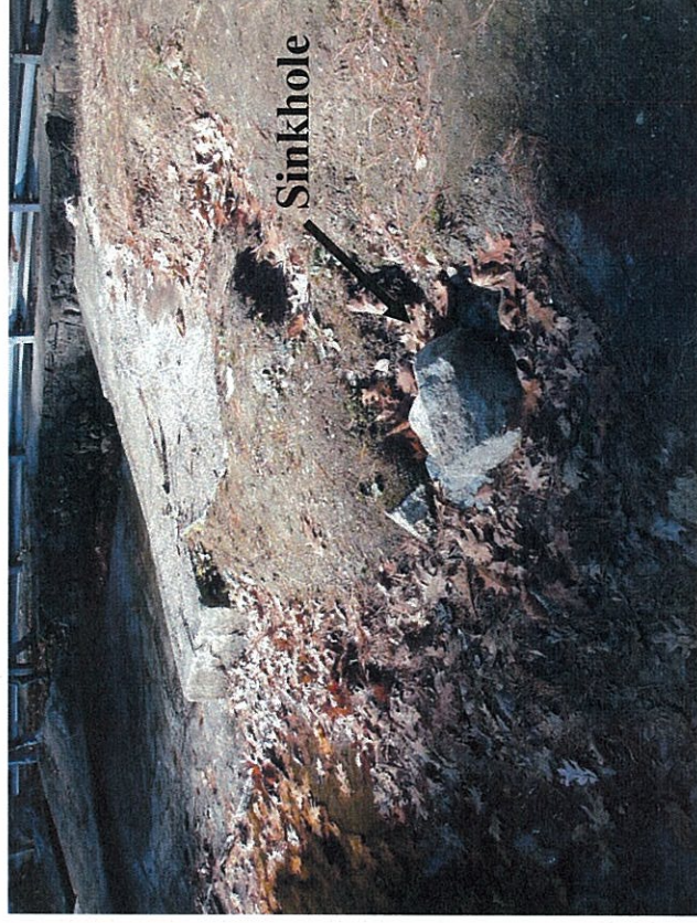
Photo 14 – Right upstream slope and crest erosion by spillway
