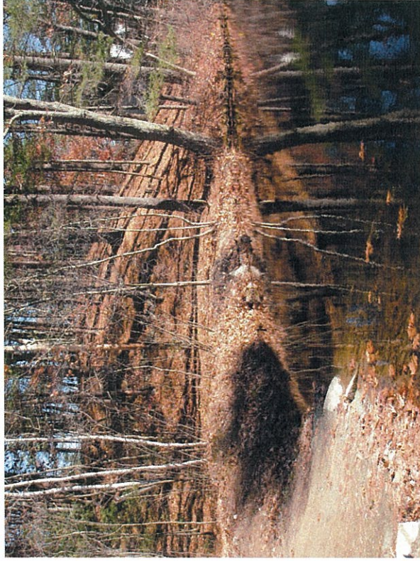
Photo 18 – Missing riprap on upstream slope
