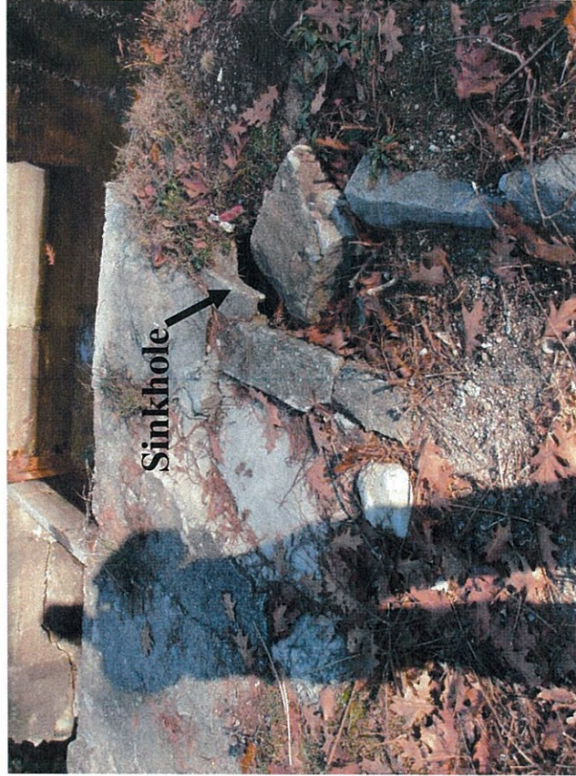
Photo 13 – Sinkhole on left side of sluiceway
