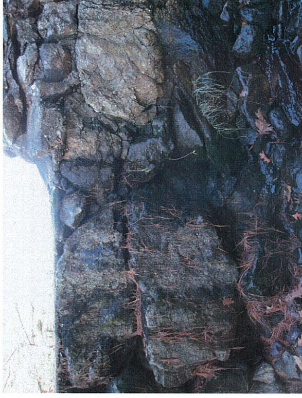
Photo 19 – Missing stones from downstream masonry wall
