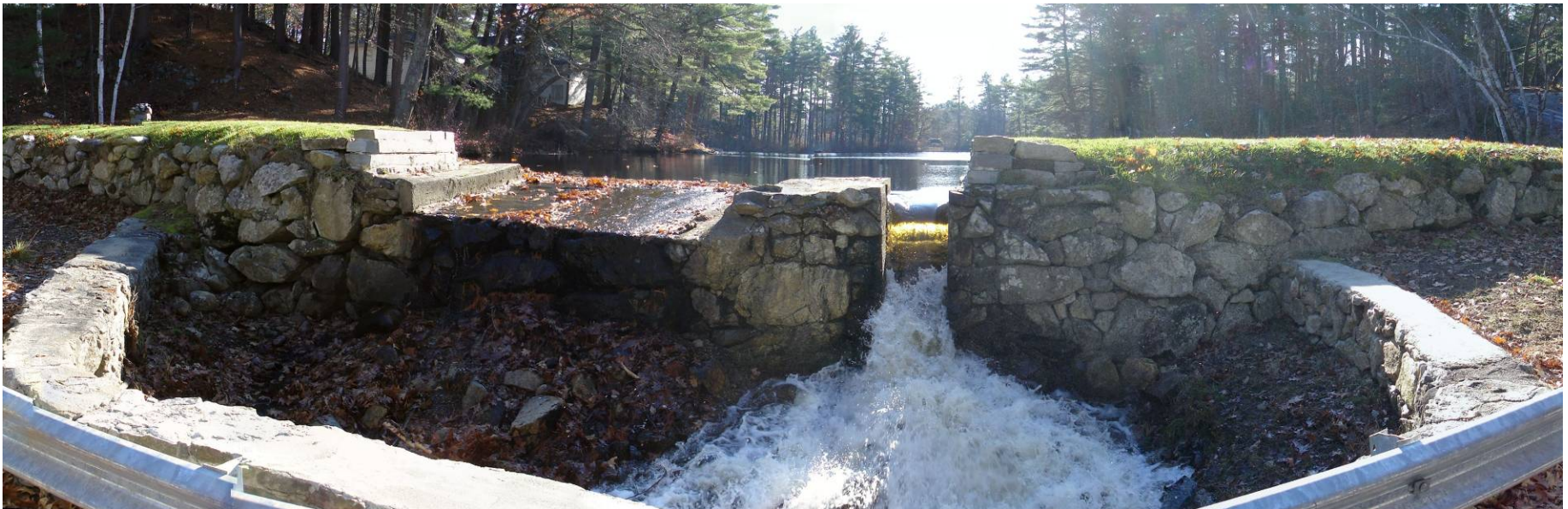
Photo 11 – Panoramic composite – Spillway and plunge pool from downstream*
