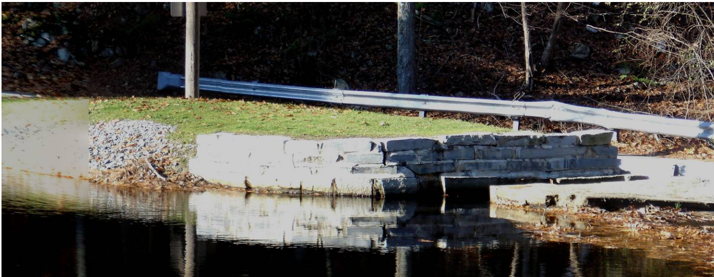
Photo 9 – Panoramic composite – Left embankment and left spillway training wall*
