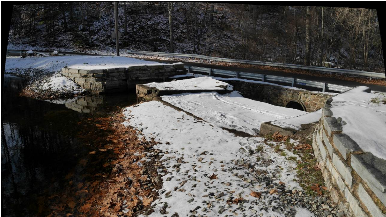
Photo 10 – Spillway and sluiceway upstream side*
