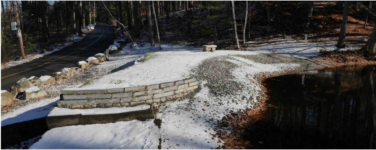
Photo 9 – Right embankment and right spillway training wall*
