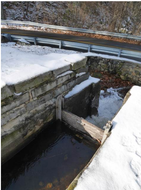
Photo 12 – Sluiceway stoplogs and new metal slots
