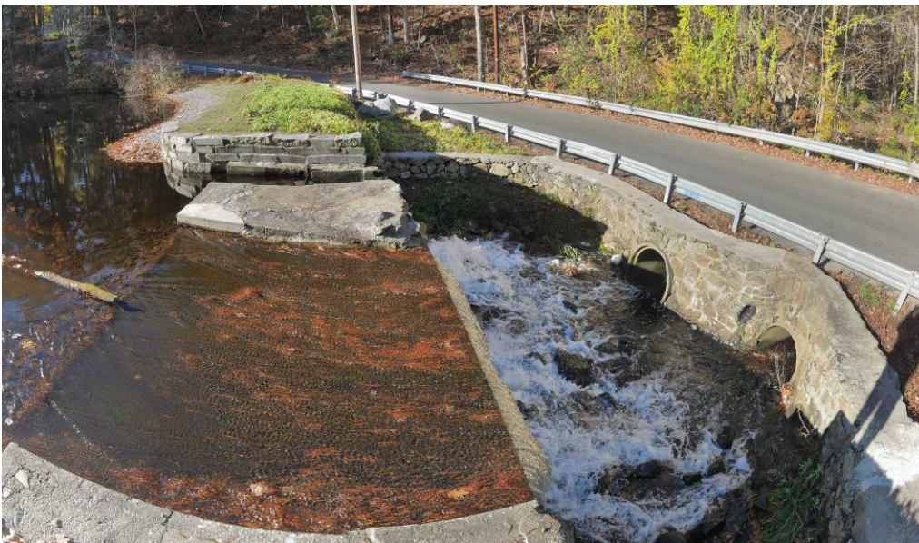
Photo 8 – Left embankment, spillway, sluiceway, and plunge pool from crest*
