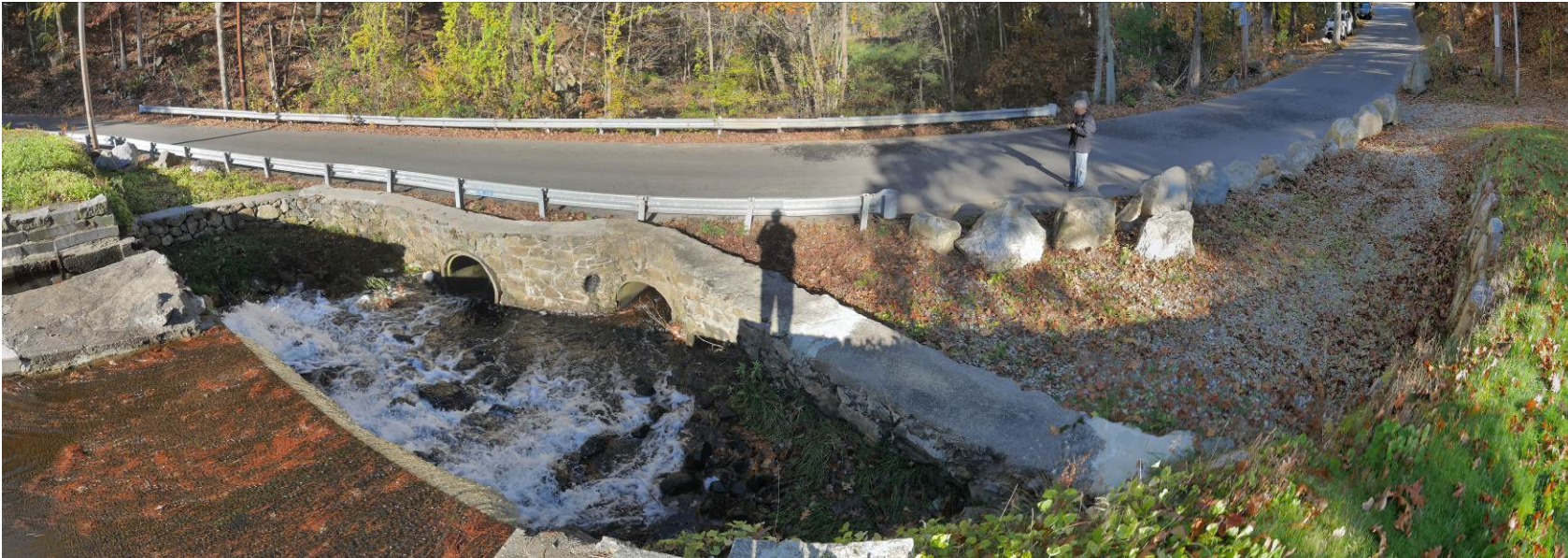
Photo 9 – Spillway, plunge pool, and downstream from right crest*
