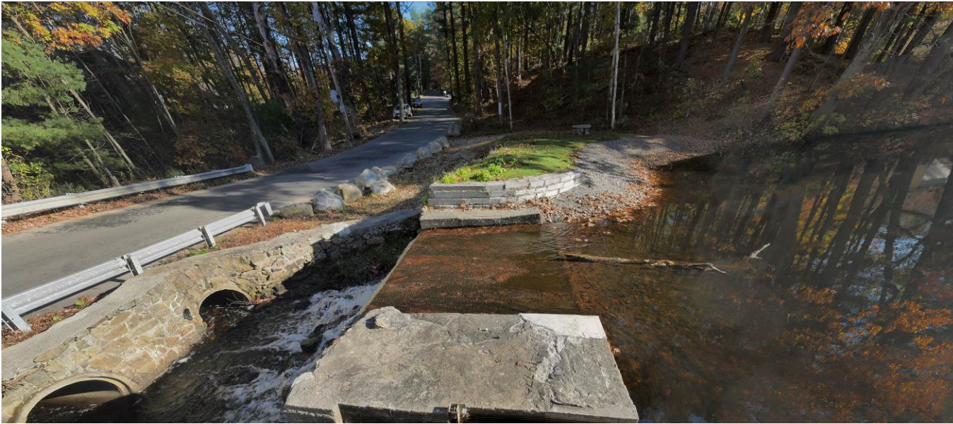
Photo 7 – Right embankment, spillway, and plunge pool from crest*
