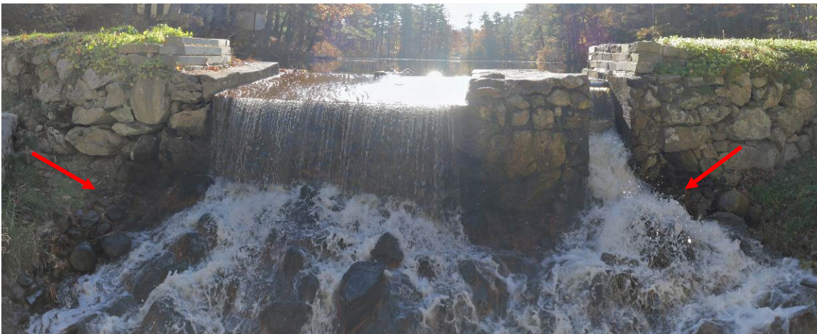
Photo 10 (left) – Spillway and sluiceway from downstream (arrows show general seepage sites)*
