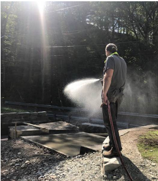
Photos 12 (upper left), 13 (upper right), 14 (lower left), 15 (lower right) – May 2021 maintenance activities – replacing spillway slab (12, 13, 14) and placement of additional gravel on upstream slope (15). Gravel also placed over auxiliary spillway. Photos from Foster's Pond Corporation website.
