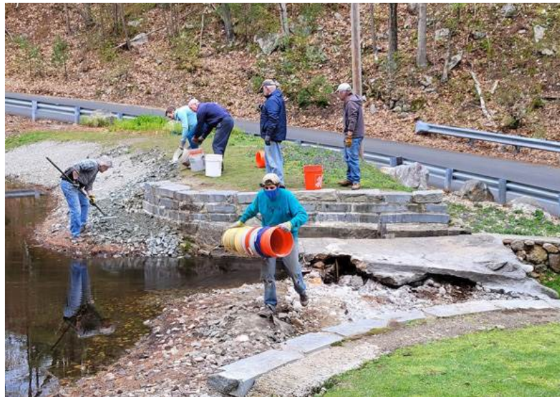
Photos 12 (upper left), 13 (upper right), 14 (lower left), 15 (lower right) – May 2021 maintenance activities – replacing spillway slab (12, 13, 14) and placement of additional gravel on upstream slope (15). Gravel also placed over auxiliary spillway. Photos from Foster's Pond Corporation website.
